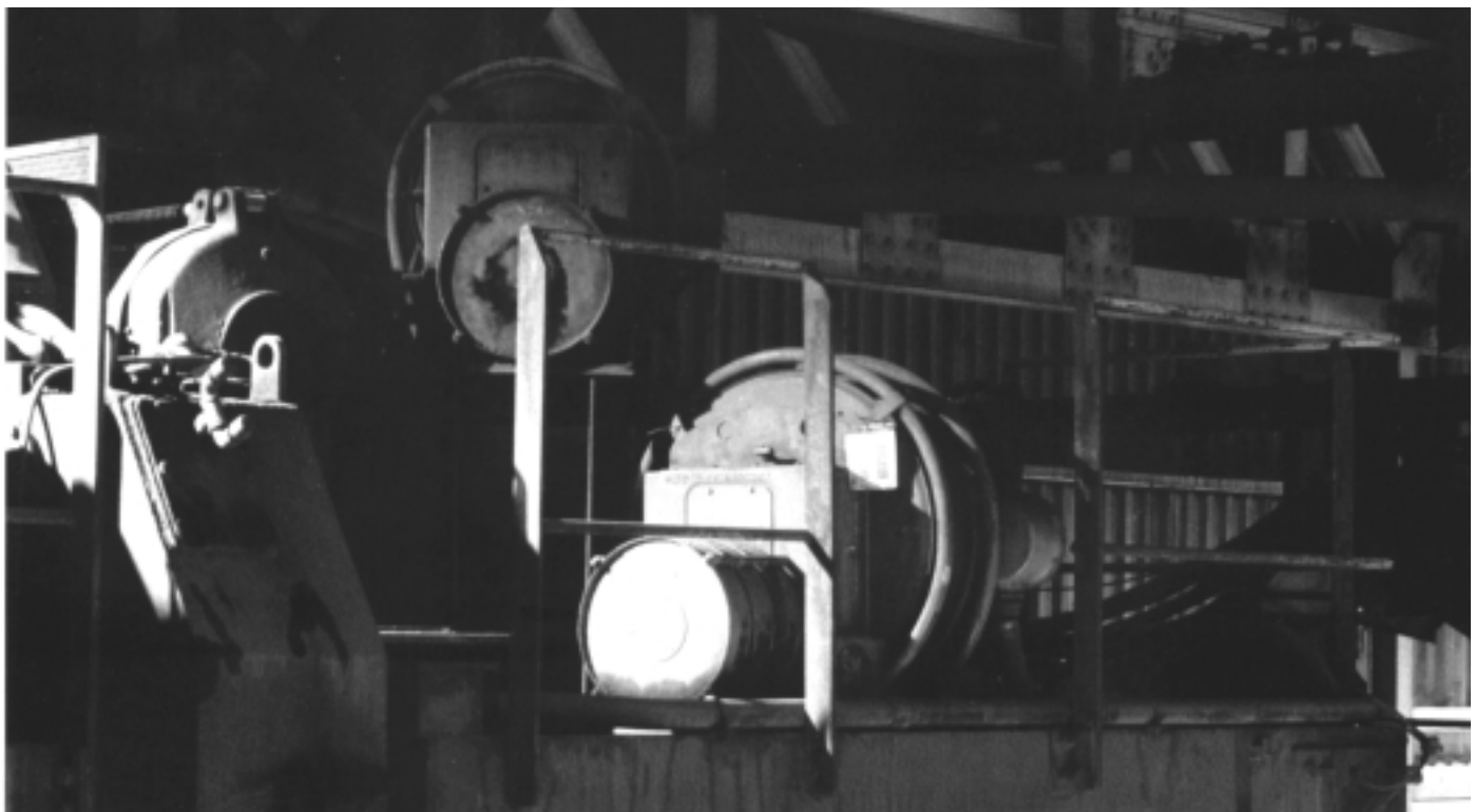
Typical SM Reel application in steel mill. Two reels shown.
